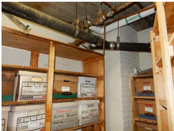
Basement of the Service Building. Credit: Willie West
